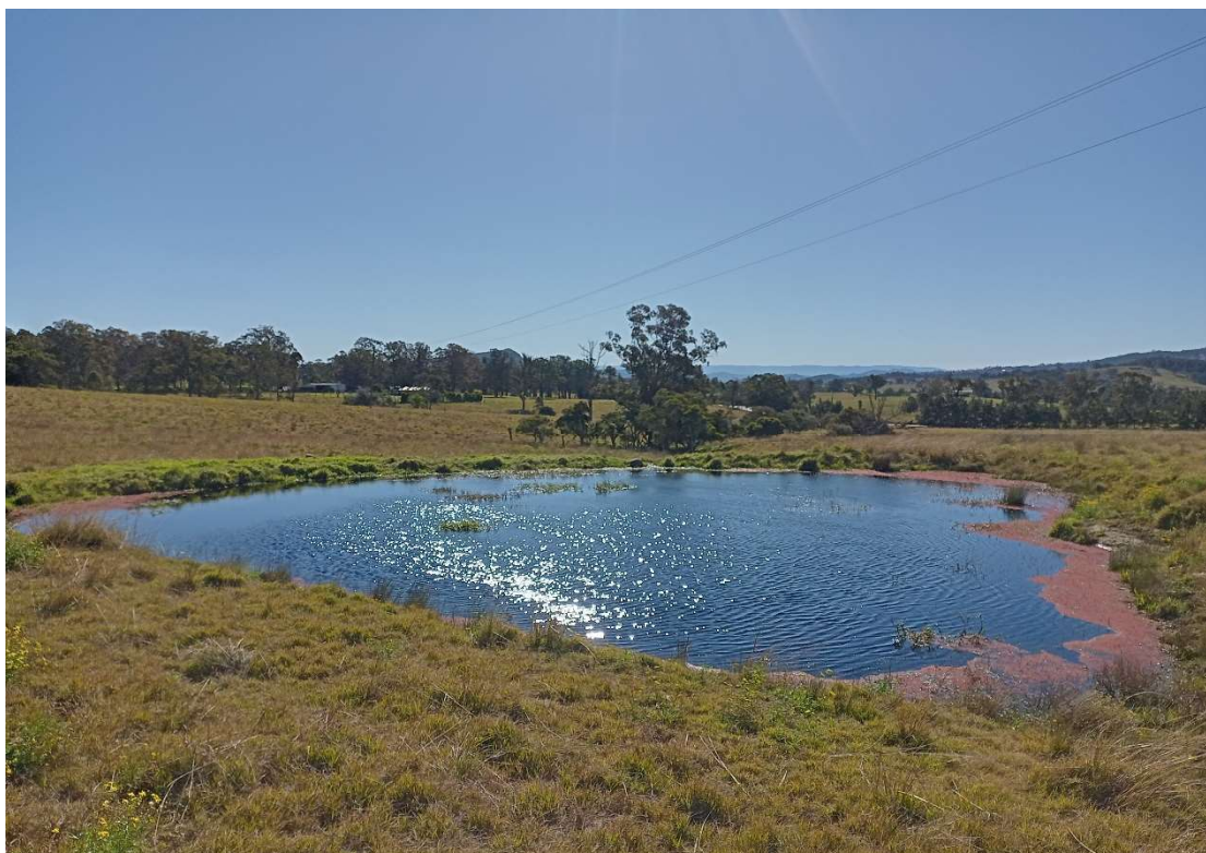
Photo 7: Looking north at Dam 5.
